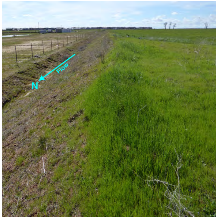
4. South parcel eastern drainage ditch
