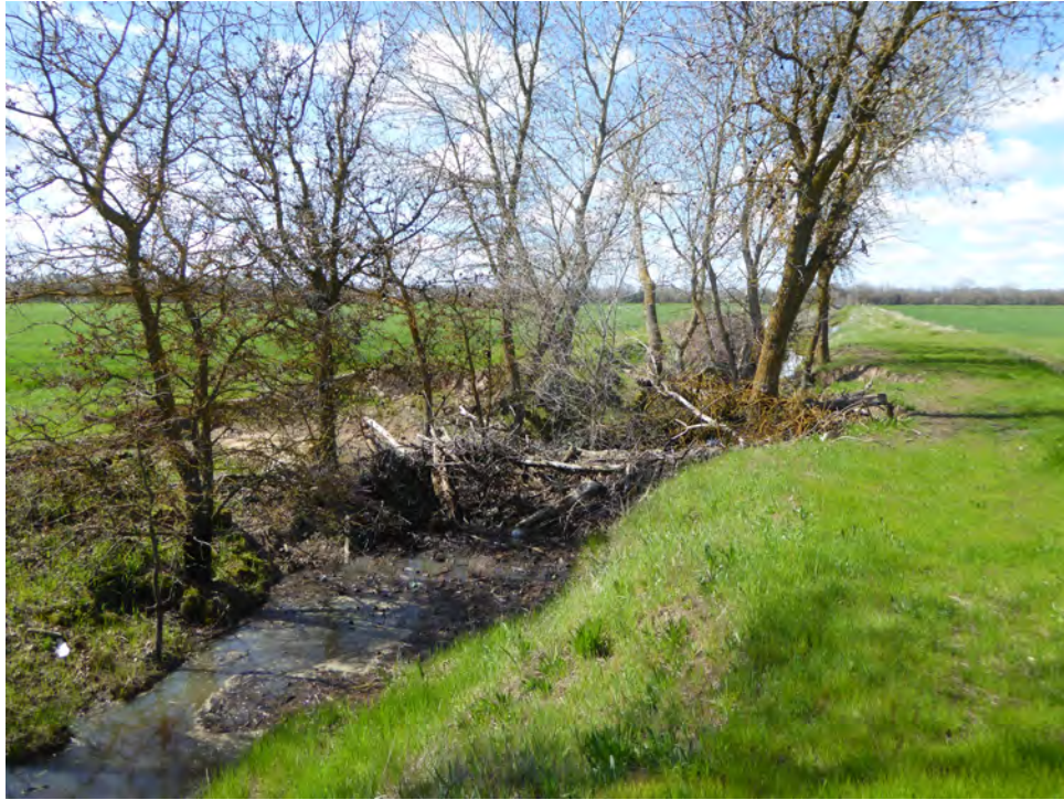
9. Debris obstruction along northern irrigation canal
